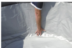
10) Smooth the liner all around the SPA to ensure a good fit.
